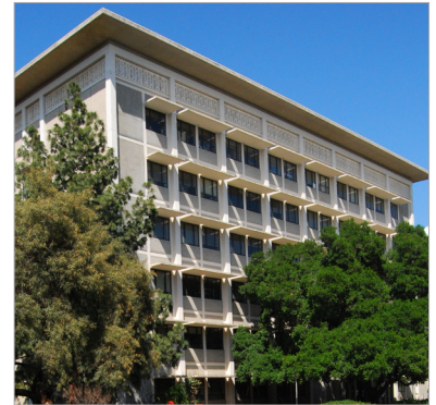
Sun control on windows (Storer Hall)
