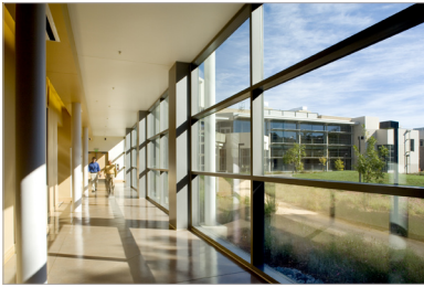
A glazed corridor continues around the Vet Med central open space, providing a gradual transition between the building and landscape and assisting with orientation
