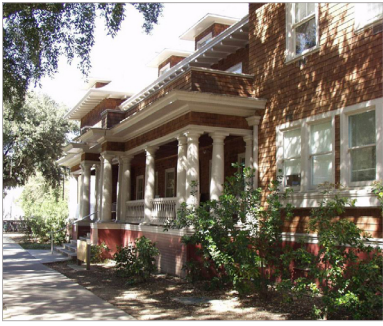
Shingle buildings such as North Hall exemplify the human-scale, highly articulated buildings of the original campus
