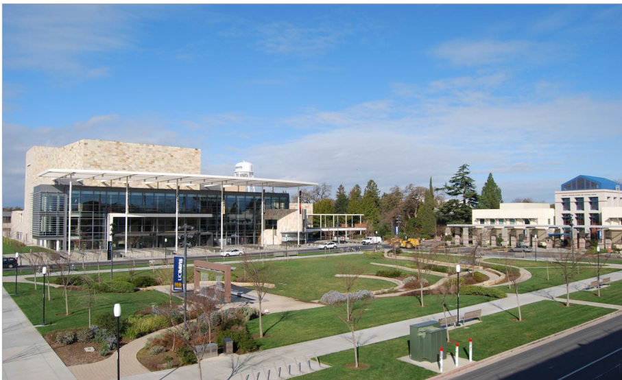
South Entry District, looking northwest into new open space, visible from Interstate 80
